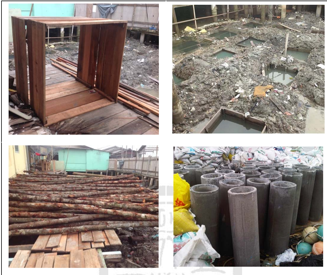
Figure 3.13 Construction site of concrete house
